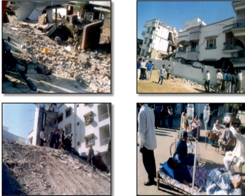
Fig. 13 : The city of Ahmadabad after Gujarat earthquake January 26, 2001 Source: Gujaratplus.com ( http://www.gujaratplus.com/news/archives/arc83.html ), retrieved on 12th October 2019.
