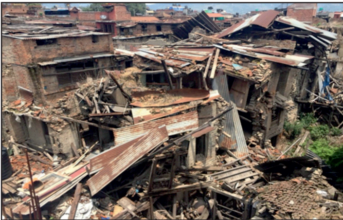
Fig. 19 : Damage to buildings during earthquake in Nepal. Source: - https://www.fatfacefoundation.org/blog/2017-09-04-nepal-earthquake-2015-update , retrieved on 20th October 2019.
