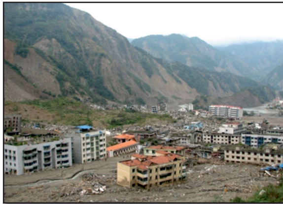
Fig. 16 : Image of the town of Qushan, Beichuan County, China after 2008 Earthquake.
