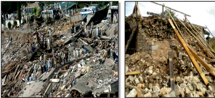
Fig. 15 : Image of Balakot (PoK) after the earthquake and collapsed stone masonry building.
