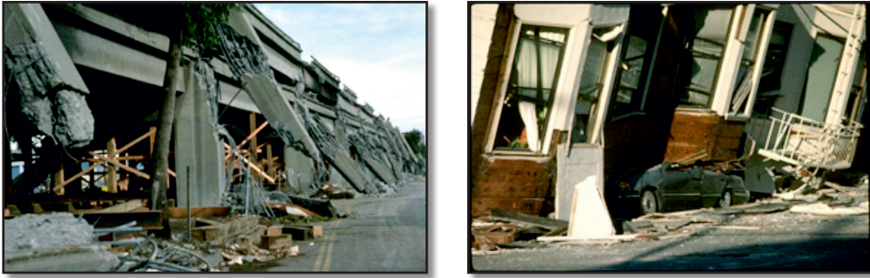
Fig. 8 : (a) Collapse of the building due to the earthquake in Oakland (b) consequences of Loma Prieta earthquake in San Francisco (Anderson, G., 1997)
