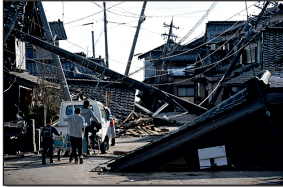
Fig. 21 : Damaged houses in Suzu, Japan
